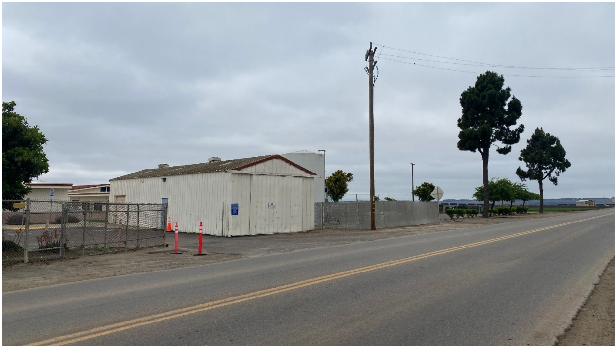
Photograph 10. Barn-like building located in maintenance area in eastern portion of Bonita Elementary School campus, view northwest.
