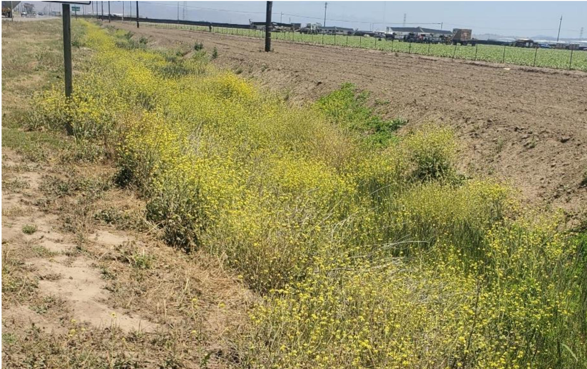
Photograph 2. Photograph of the existing ditch along the south side of State Route 166, facing southeast. June 28, 2023.
