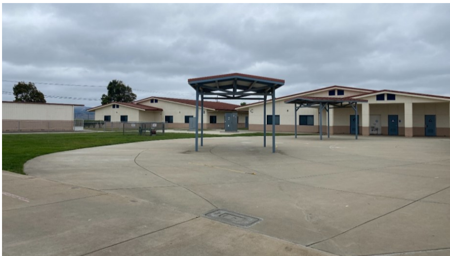
Overview of the buildings surrounding the Bonita Elementary School quad, view northwest.
