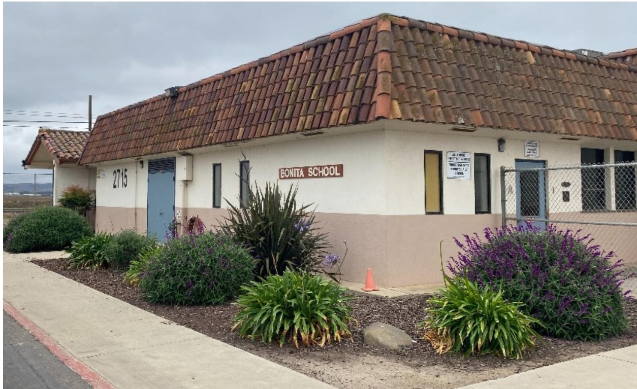
Photograph 7. North and east elevations of Bonita Elementary School Kindergarten Building, view southwest.
