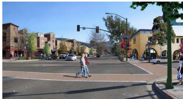
This is what the intersection of H St. and Chestnut Ave. could look like in 10 yrs.
